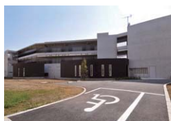
外観(北側) View from the north side
